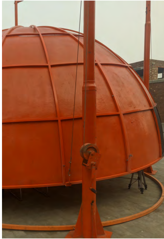
Figure 11. The steel wire loops through the pole's pulley and attaches to a carpal's baseplate.
