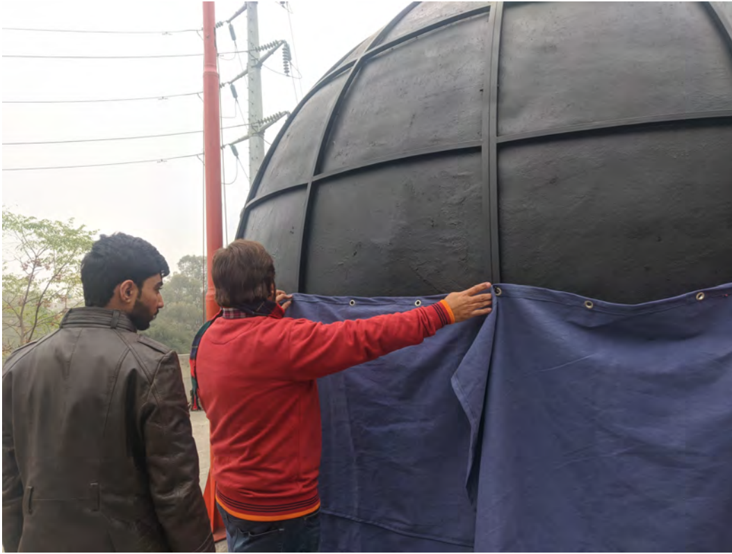
Figure 50. Hang the tarpal on the hooks outside.
