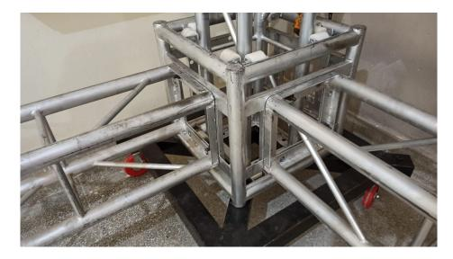
• Hang the pulleys with the vertical columns (8 feet) and tie the chains with the square structure. With the help of four team members, pull the truss to its height.
